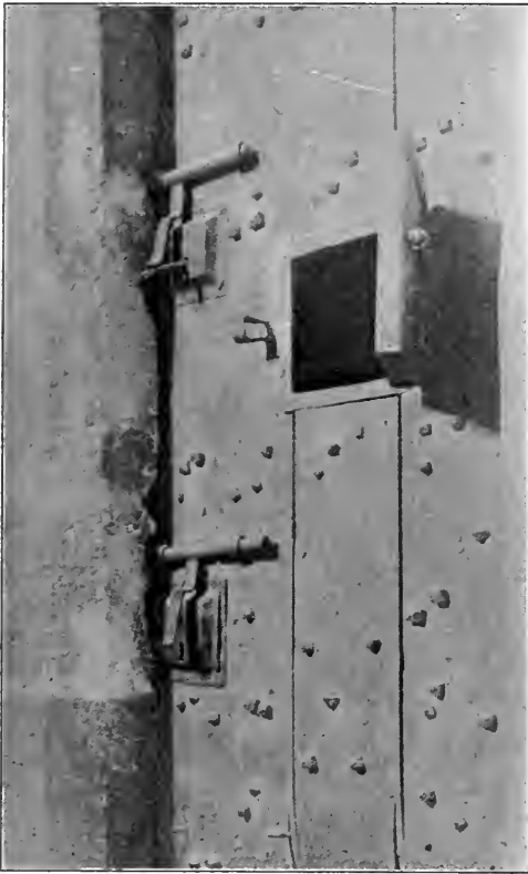
FIG. 22.—ANCIENT LOCKS, BOLTS AND PEEP-HOLE IN THE PRISON DOOR. Château of Langeais.
